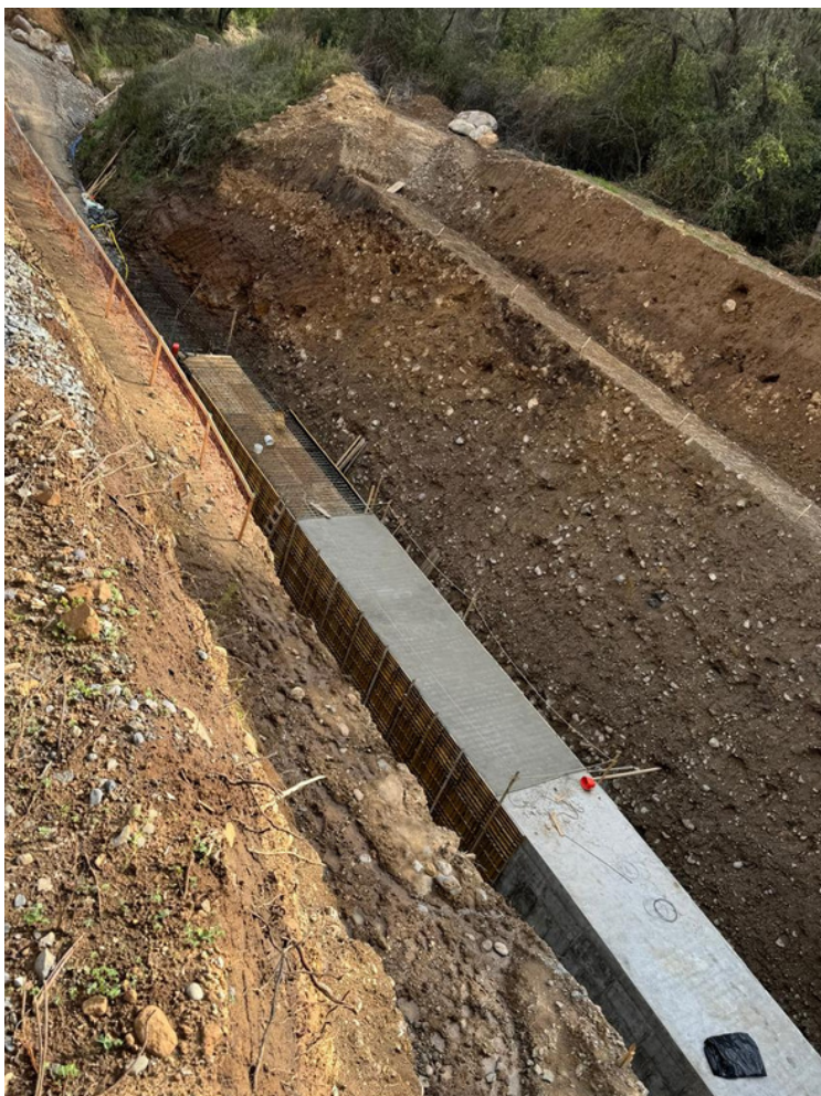
TUNEL LA GREDA 70% avance
